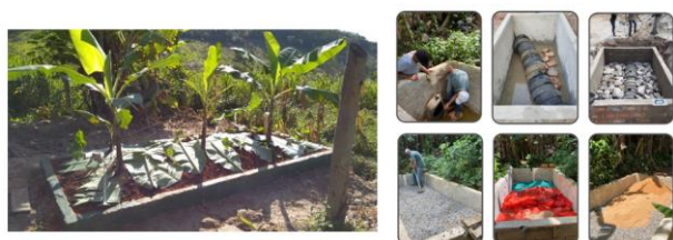
Figure 7. Evapotranspiration System (TEvap) using concrete chambers filled with stones, tires, sand and soil that receive the sanitary sewage. Banana plants ( Musa sp. ) are responsible for nutrient absorption and water transpiration.
