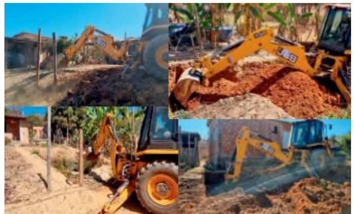
Figure 5. Construction of the septic system using an excavator
