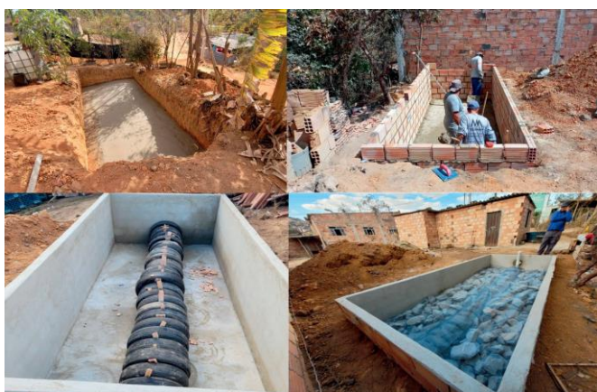
Figure 6. Evapotranspiration System (TEvap) construction process.
